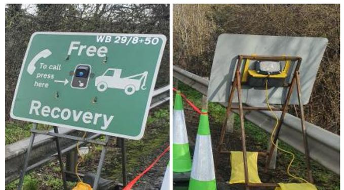
The CCT can also be deployed as an emergency call point for road users to summon vehicle recovery services. Having an accident or breakdown in the middle of road works can be a worrying time so having a readily accessible emergency call point provides vital comfort and reassurance to road users. At the push of a button, they can speak with someone, explain their emergency situation and get reassurance that help is on its way.
