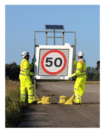
Dynamic Speed Signs have changed this. Using digital technology, the new signs can automatically change to display 40, 50 or 60 mph according to the works programme. This removes the need for operatives to physically change signs which keeps them safe. It also allows traffic to flow freely at 60 mph when works are stopped, minimising disruptions and improving journey times.
